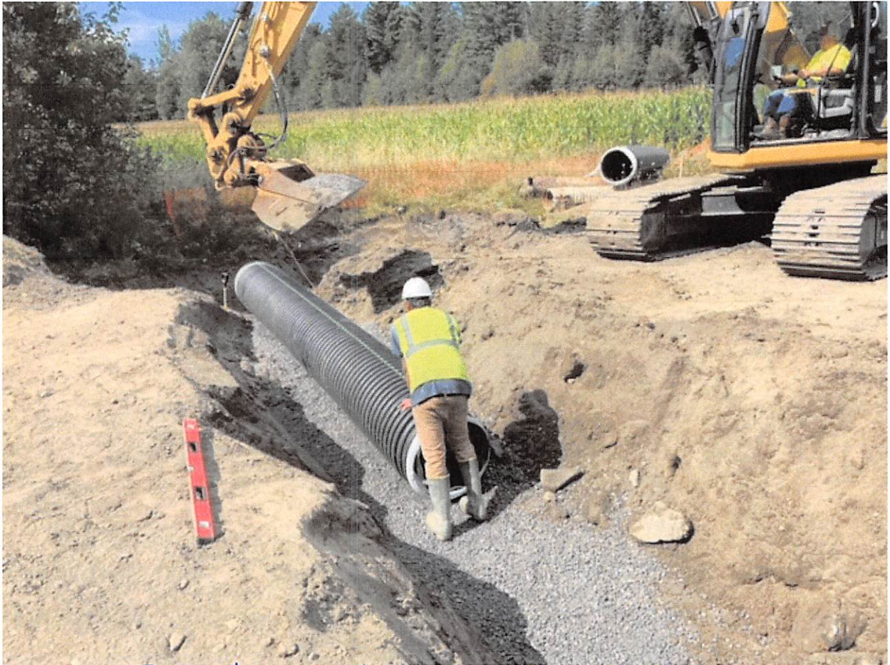
South Site Work in Progress
